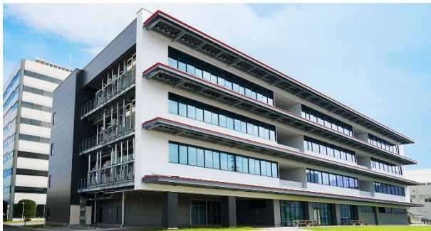
SUSTIE ZEB Test Facility
